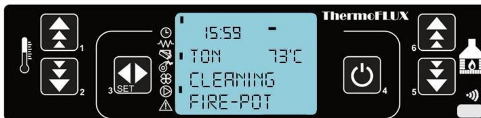
When cleaning phase is finished, boiler will continue to work and power will be set on power chosen before.
